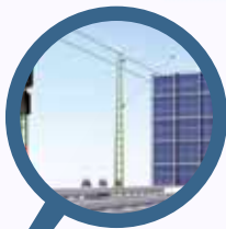
Cables for catenary
