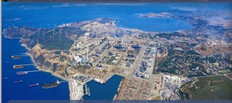
Socar - Star Refinery
